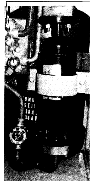
Stop valve at the accumulator-receiver outlet side
