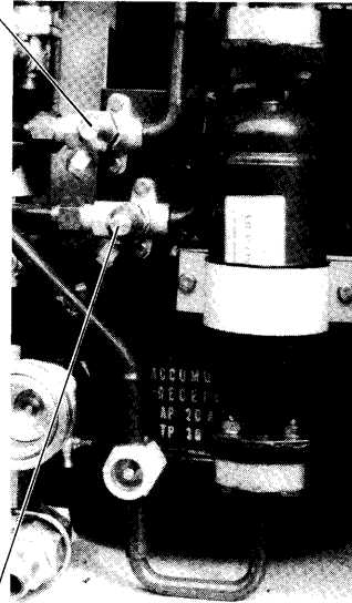
Stop valve at hot gas bypass
